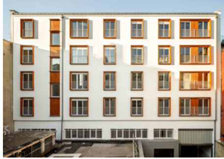
Figure 12. Conversion of post office building into housing, Bien Urbain Atelier d'architecture.
