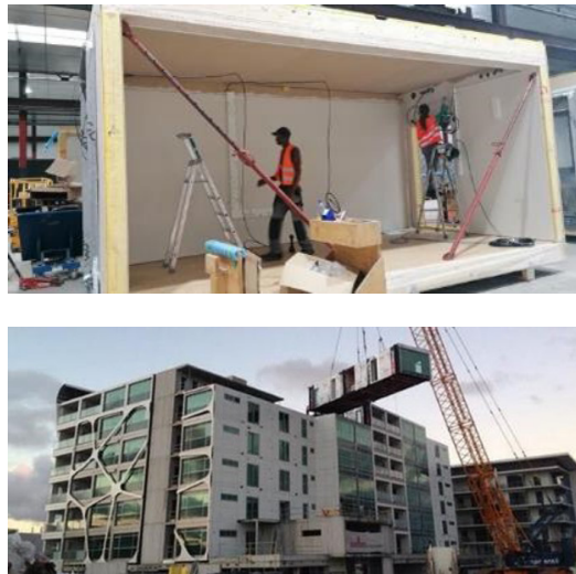
Figure 5. Off-site construction, from factory to construction site © Aurenche, Eric, 2020.
