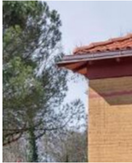
Figure 17. Cantenac Brown adobe walls
