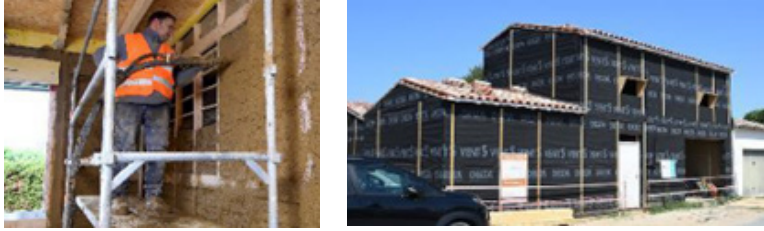
Figure 19. Process for building a single-family home with Terlian® technology
