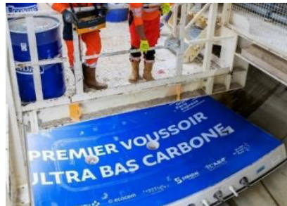
Figure 22. Keystone for the Grand Paris Express using a binder that reduces CO2 impact by 90% © Grand Paris Express, 10 février 2022.
