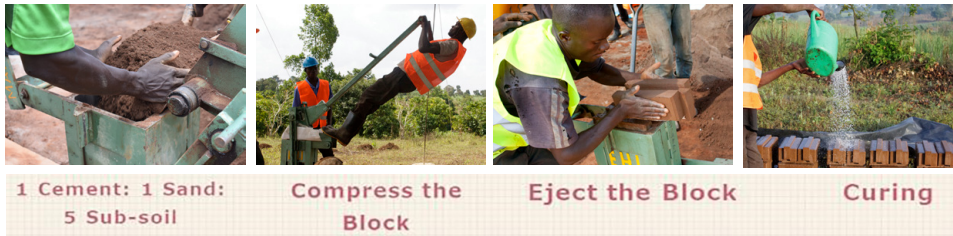
Figure 16. ISSB manufacturing process © Nambatya, Mauricio. 8-12 avril 2024.
