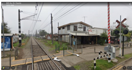
Figures 3, 4. Current state of the infrastructure, Google Earth
