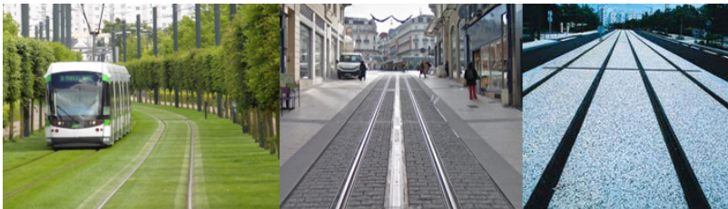
Figure 10. Types of surfacing for tramway platforms © Transport urbain
